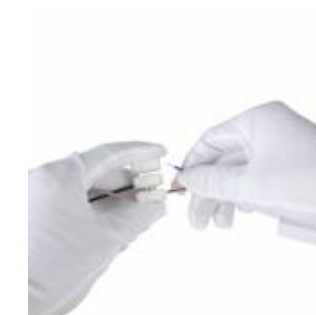
Step 3: Connect the cables of the lamp to the cables in your home.
